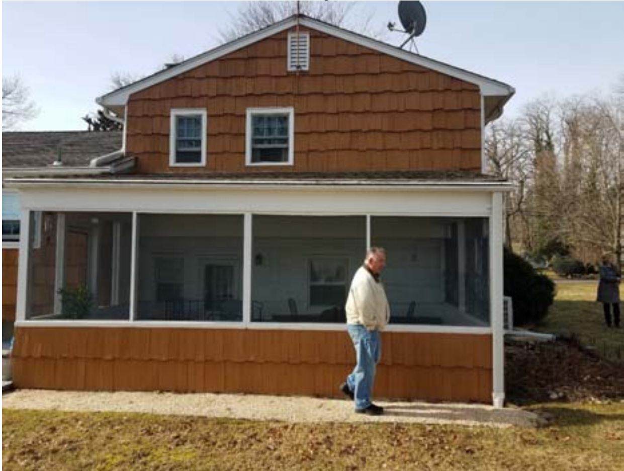
3A.20 Roof (not roof structure) comparative rating: apparently fairly good
